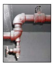
Does the 40-foot-long (12.2 m) trapped branch line described below require a low point drain? Assume the sprinklers are attached directly to fittings on the branch line, and the pipes are joined with grooved fittings that add no extra water carrying capacity.
